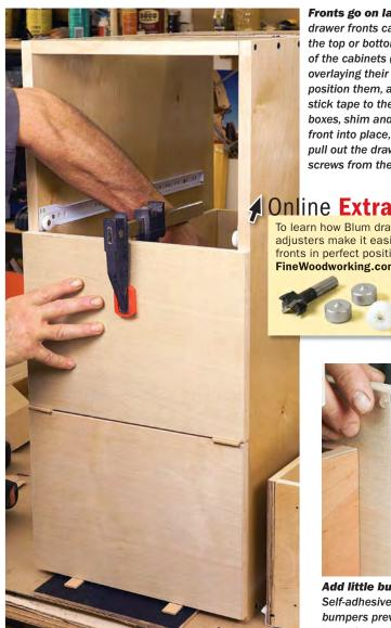
Fronts go on last. The drawer fronts can overlap the top or bottom edges of the cabinets (as well as overlaying their sides). To position them, apply doublestick tape to the drawer boxes, shim and press each front into place, and then pull out the drawers to drive screws from the inside.
