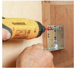
**Attach the bracket.** The bracket attaches to the cabinet back. It will work better if the back is ½ in. thick vs. the usual ¼ in.
