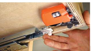
Click the slides into the locking devices. Pull the sliding sections forward to click them into the locking devices. The drawer is installed.
