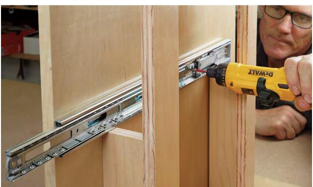
Same approach as before. Use a combo square to lock in the inset from the front edge of the cabinet, and a self-centering bit to drill pilot holes before driving screws. The cabinet part of the slide has an extra section, which you'll slide fore and aft to expose the screw holes.
