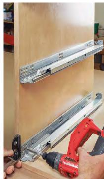
**Bottom two pairs.** Rotate the supports to install the middle pair of slides. The lower pair goes against the cabinet bottom.
