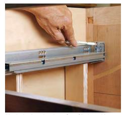
Mark the bracket location. Sit the cabinet slide on its vertical supports, push it back into the bracket, and mark the screw locations.
