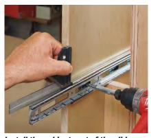
Install the cabinet part of the slide. Again, use two-part supports to position the slides as you attach them to the cabinet.
