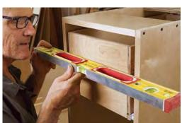
Use a straightedge to make sure each drawer is installed squarely, with its front face even with the cabinet or slightly inset. The slides have alternate screw holes for adjusting the slide positions.
