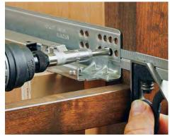
**Attach the slides.** Use that combo-square setting to locate the front edge of the drawer slide. It gets attached to a post in this piece, but in a face-frame cabinet there would be another filler strip up front for attaching it.
