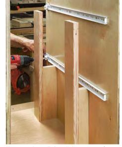
Next one down. To install the next set of slides, rotate the supports to use the lower parts. Install these slides the way you did the upper ones, using a combo square to set the inset and a self-centering bit to drill pilot holes.
