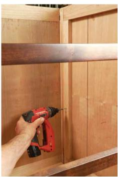
**Add filler strips.** Mill strips to fill the offset between the inside edges of the face frame and the cabinet sides, and then screw them into place.
