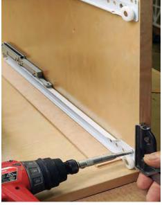
Bottom pair. These go at the bottom of the cabinet. There is a bump under their front edge, so place a 1/8-in.-thick spacer just behind it. This will keep the slide level and ensure that the drawer part won't rub on the cabinet.
