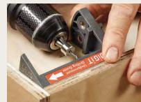
Same guide works up front. Tilt the guide to line it up for drilling angled pilot holes in the front of the drawer box.
