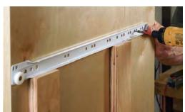
do it. Use a self-centering bit to drill pilot holes for the screws so the slide doesn't shift. Start with the first screw, recheck the inset, and then drill and drive two more screws.
